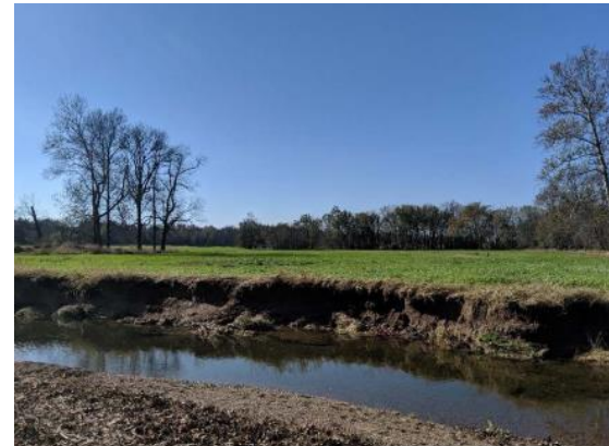
Pre-construction 6-foot-high eroding bank with historic floodplain layer under legacy sediment
