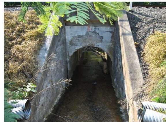
Typical culvert within the Borough
