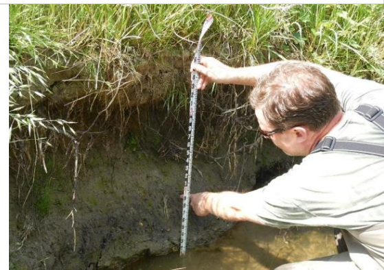
Pre-construction eroding bank with historic floodplain layer under legacy sediment
