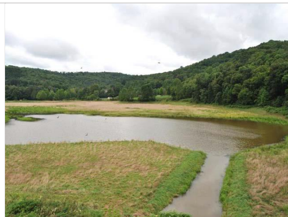
Overview of former Duke Lake after the dam was lowered
