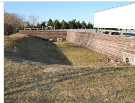
Commercial basin for potential retrofit
