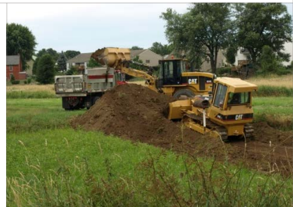
After – Sediment removal from the Forebay
