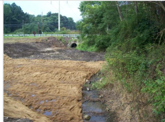
Floodplain restoration during construction
