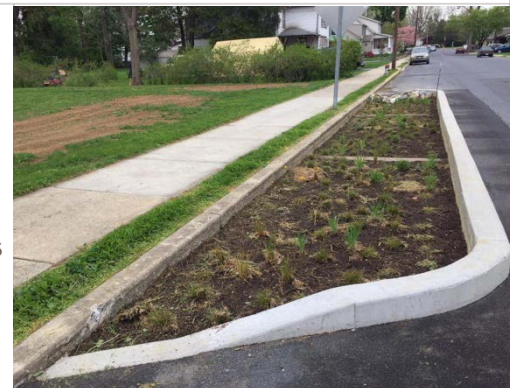
Bump out with installed raingarden along Locust Street
