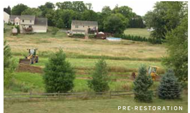
Sediment build up is being removed from the pretreatment settling basin.
